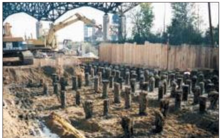
Remediation of a kerosene spill below a pile supported foundation
